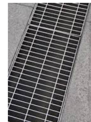
Galvanized grate drain
